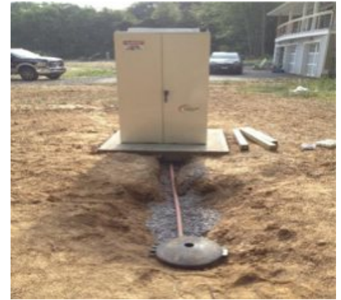
Hydrogen Tank Connected
